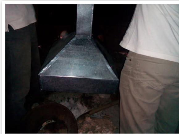
Chimney flue with smoke chamber above existing furnace.
