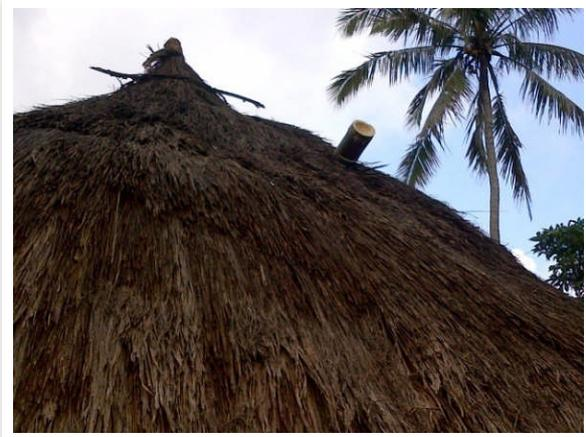
Chimney extension made from bamboo.
